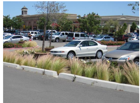
Figure 1-1. Bioretention facilities infiltrate most runoff (above) and can be an attractive landscape amenity (below).
